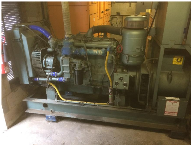
Photograph 2: Diesel generator located on the roof.
