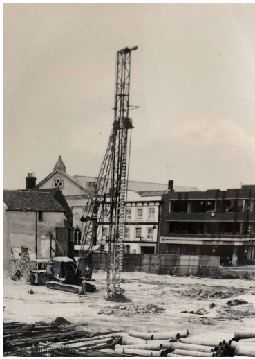
Figure 10: Piling Rig construction Early Phases of Kennet Centre
