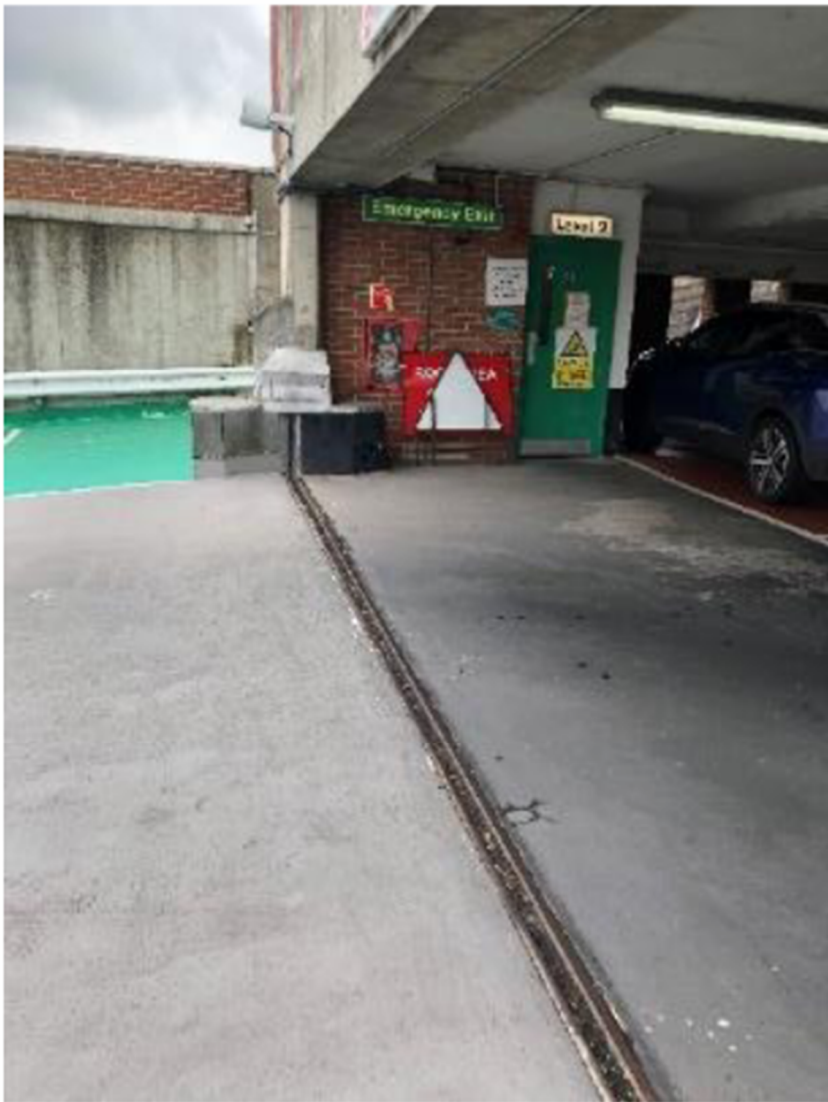
Figure 38 Photo showing movement joint and separate strucures of MSCP and former Sainsburys.
